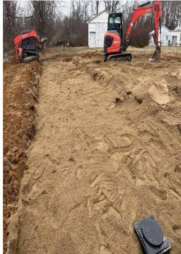
Filled in Sand Bed
