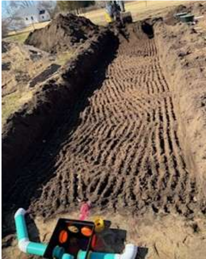
Raking of Sand Bed
